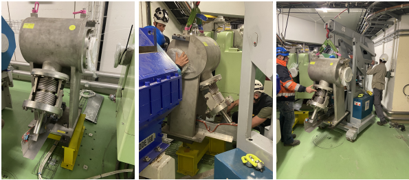
Fig. 21. Removal of Fig. 1(b)-type beam stopper from CERN transfer line.
