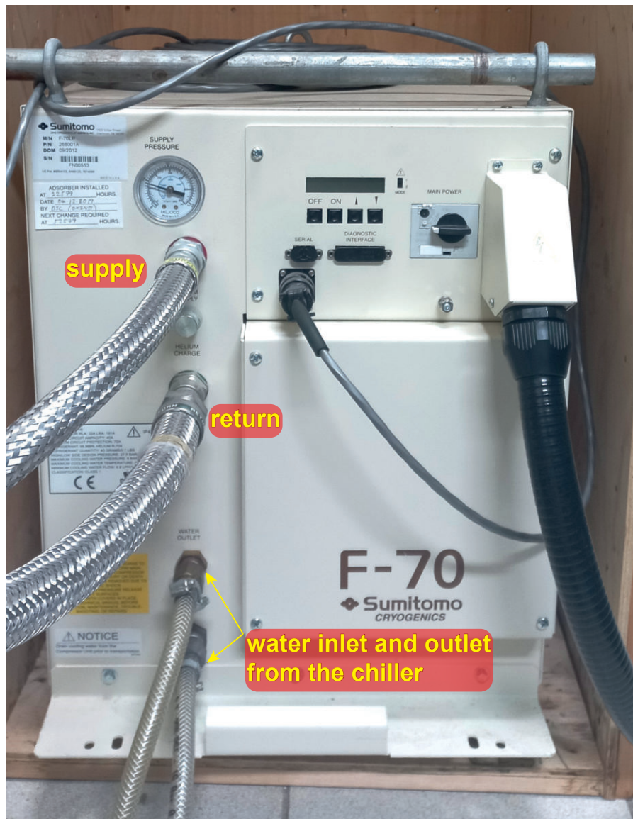
Figure 3.9: F-70 Sumitomo compressor showing the supply and returns ^4\text{He} lines and the water inlet and outlet lines from the chiller to cool down the compressor during its functioning.
