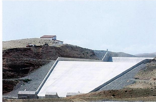
Figure 3 Ogee spillway of Aghchai dam
