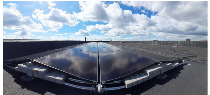
Figure 5: Photograph of a section of the installation showing the delta east-west configuration.
