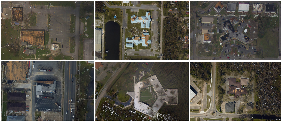
Figure 6. Examples of significantly damaged facilities (first column—fire station (top left) and pharmacy (bottom left), all the rest are hospitals and clinics. Source: NOAA, 2024.
