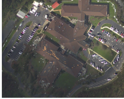
Figure 5. An example of the facility damage to which was considered minor. Intact parking area and present accessibility indicate that this facility is fully operation despite visible roof damage. Source: NOAA, 2024.
