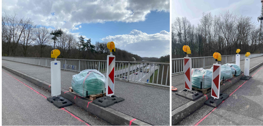
Figure 5: The initial additional mass at the quarter point (left) and three additional masses at the center of the bridge (right).
