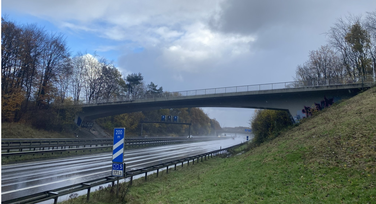
Figure 1: North view of bridge 'Vahrendorfer Stadtweg'.
