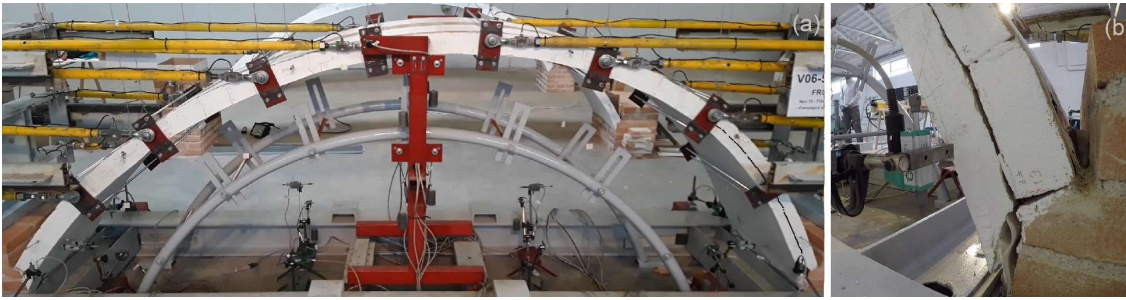
Figure 15. Configuration of sample vtRI+ at the incipient collapse, evidencing the partial detachment of the pre-existing plaster layer from the masonry, on the right side: (a) global view and (b) detail at the right skewback.
