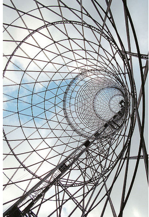
(b) The grid shell of the Shukhov Tower in Moscow, whose sections are doubly ruled. The image has been adapted from Wikipedia.
