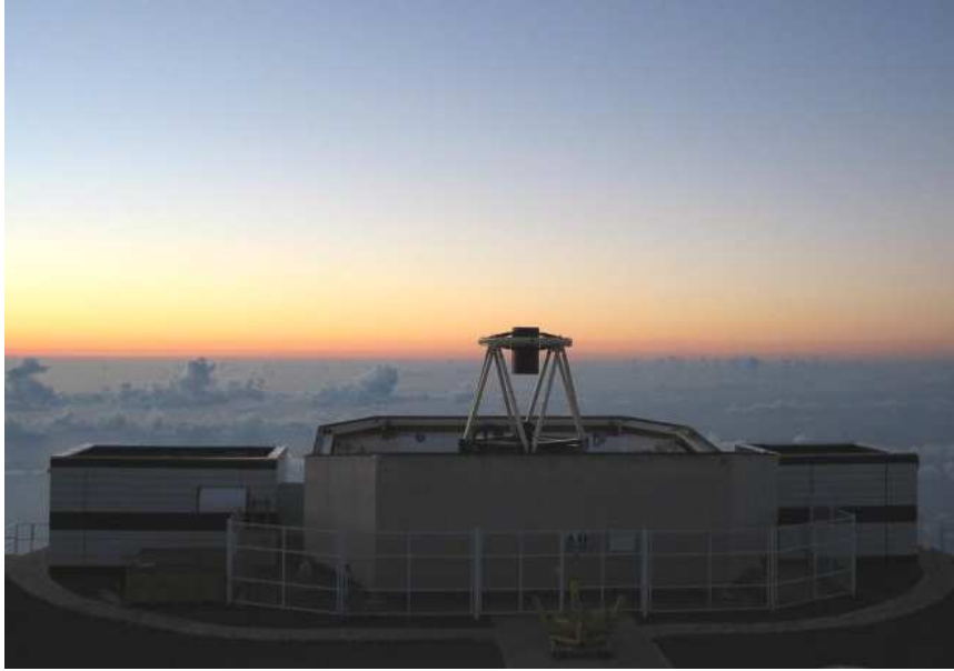
Fig. 1. The Liverpool Telescope at Roque de los Muchachos, La Palma, Canaries is a 2-m fully robotic altitude-azimuth design telescope. Fully openable enclosure and the slew rate > 2^\circ/\text{s} enable the start of observations in less than a minute after the GRB alert.
