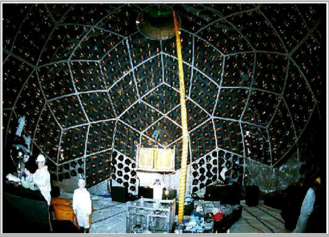
FIG. 36. View of the internal volume of the KAMLAND sphere during the central detector installation. A modular styrofoam raft is used as a platform for workers. The installation begun from the top of the sphere and moved down, as the water level in the sphere was reduced. PMTs, black shades, acrylic plates, monitoring LEDs and cables were mounted in place for each level before lowering the water.
