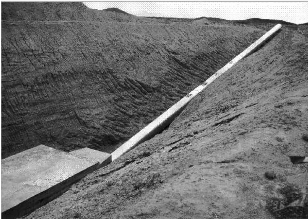
FIG. 21. The PALO VERDE underground laboratory at the time of construction (Fall 1996).
