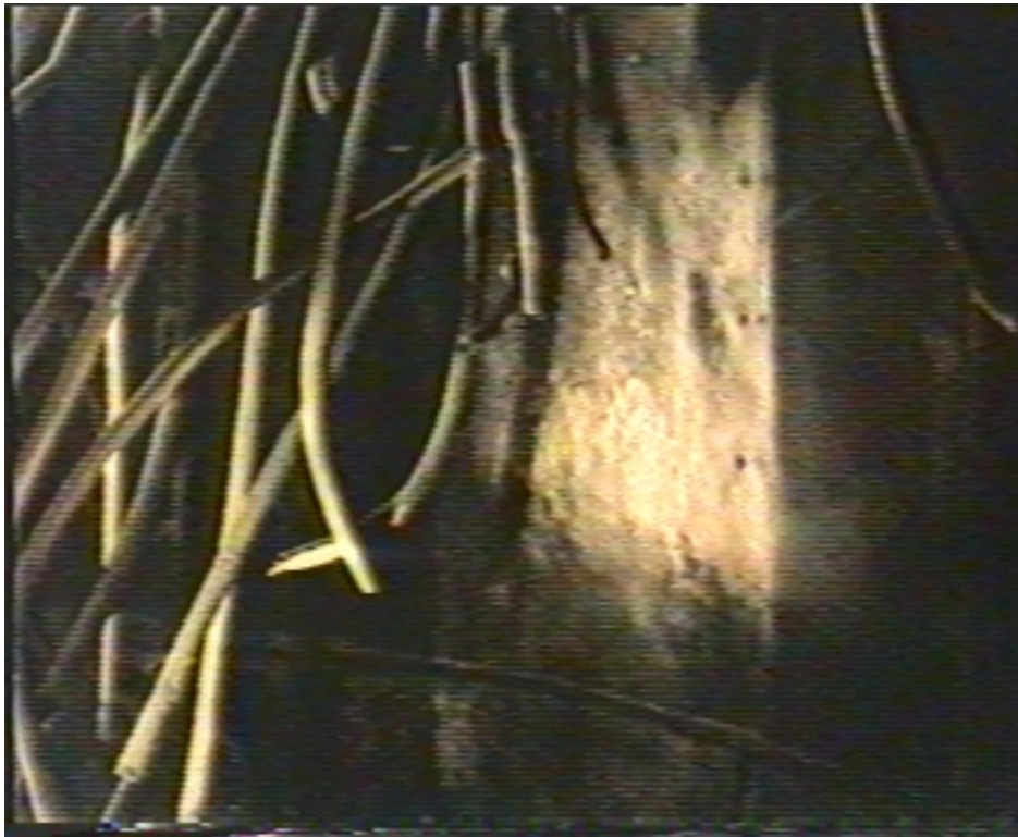
Fig. 2. A fragment of the internal surface of the reactor shaft.
