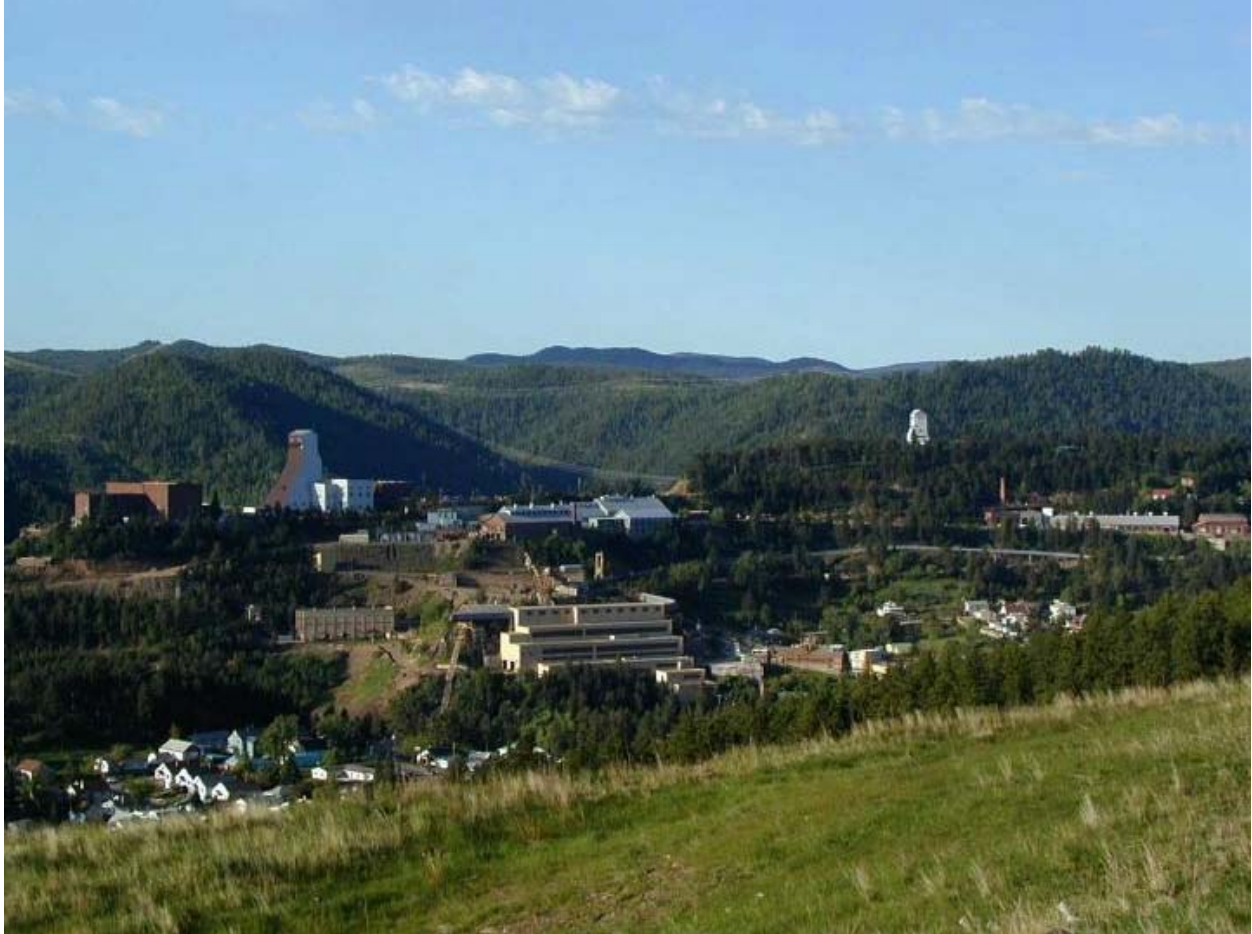
Figure B.2: A view of the Yates (left) and Ross (right) headframes. The distance between the two shafts is approximately one kilometer. These shafts/hoists provide the principal access to the 4850 ft level. In the facilities development plan, the Ross and the No. 6 Winze provide scientific access to all laboratory levels. The Yates would normally be used as the excavation shaft (together with the No. 4 Winze to reach the 7400 ft level), but could also be dedicated to megadetector construction, to give this experiment maximum access. See Section E, Figure 3, for the corresponding underground view, showing planned laboratory excavations.
