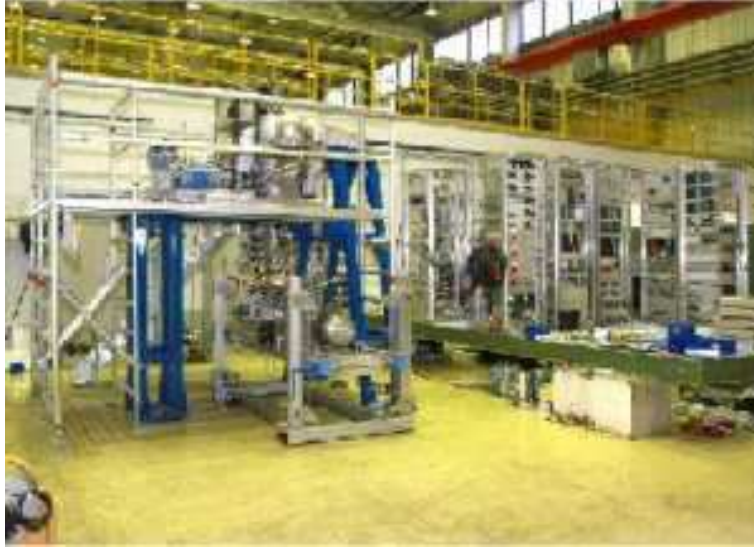
Figure 9: Polarised Internal Target installation at the off-beam position. The blue pillars on the left that support the bridge on which the ABS is mounted, exactly mimic the D1 and D2 magnets of ANKE.
